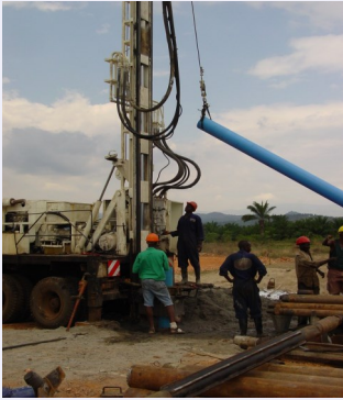
Installation of borehole casing CICR Burundi, Rumonge
